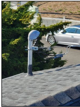
There is an overhead service drop noted.
