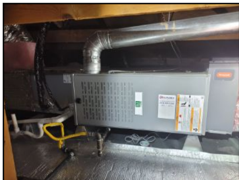
Furnace was in overall normal operating condition however we recommend contacting a licensed HVAC contractor to repair/ service the unit prior to normal use.
