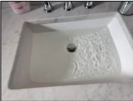
Drain showed signs of minor back up at the time of inspection recommend repairing/ replacing as needed.
