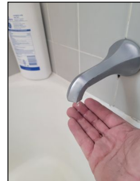
Tub faucet was not properly operating both shower head/ spout were operating at the same time recommend contacting a licensed plumber to repair/ replace as needed.
