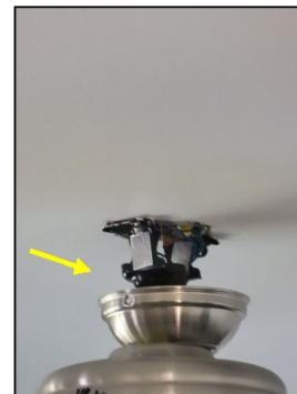
The ceiling fan canopy was not properly installed, recommend repairing/ replacing as needed.
