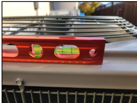
Air Conditioning mounting pad not level; this may shorten motor life. Suggest leveling pad or unit.
