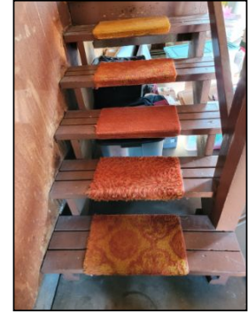
Recommend adding riser cover to improve general safety.
