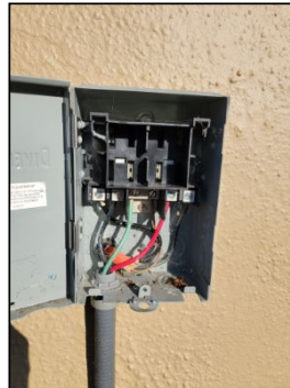
Exterior Sub-Panel (Cover off)
