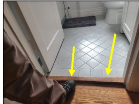
Threshold type at the hallway bathroom was noted as a potential trip hazard, we recommend improving/ updating as needed.
