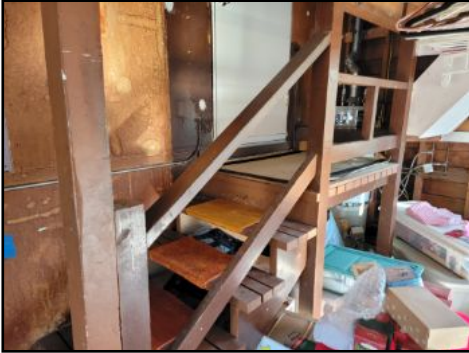
Balusters are over 4 inches apart, dangerous to children repair/ replace as needed.
