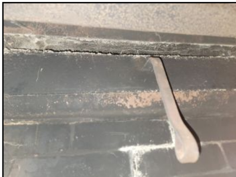
Recommend replacing damaged clean out cover as needed.
