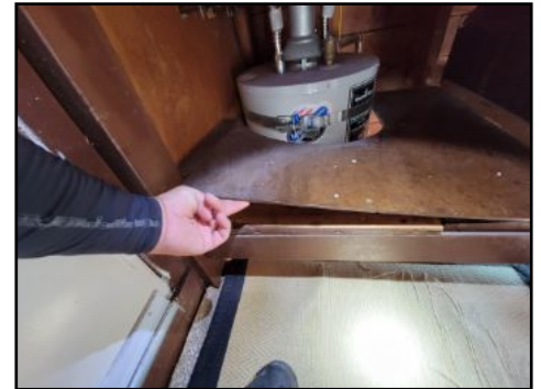
The upper landing was poorly installed or installed in a substandard manner (built around water heater/ landing does not have proper measurements), recommend improving/ replacing as needed.
