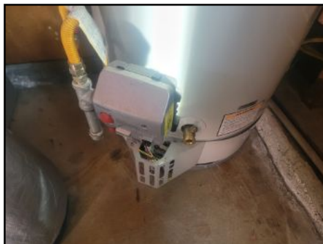
Recommend adding a drain pan to the water heater as needed.
