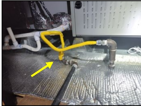
Gas shut off valves were present and functional.
