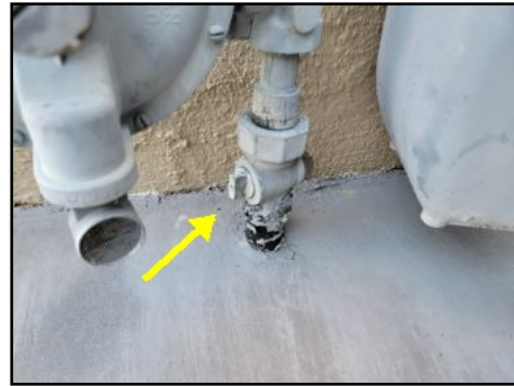
Main gas shut off valve.
