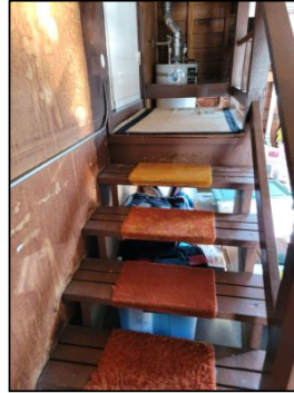
Grab bar/ railing was missing and/ or nonconforming this is noted as a potential safety hazard/ concern. We recommend contacting a licensed professional to repair/ improve as needed.
