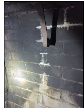
Efflorescence observed within the fireplace; often a sign of water infiltration/exfiltration and can be a precursor of masonry deterioration.
