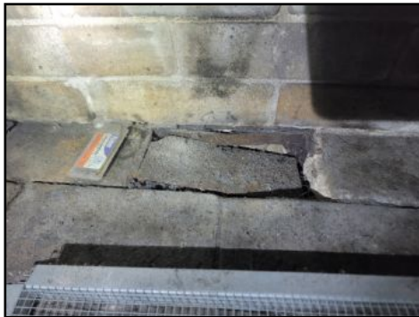
Recommend replacing damaged clean out cover as needed.
